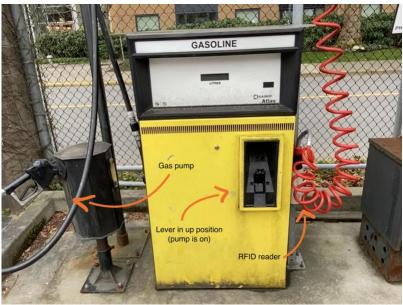
3. Once you've done that, take the RFID reader (red cable in right hand side – see Figure above) and hold it over the RFID chip inside the truck's gas cap. You should hear it beep twice.
