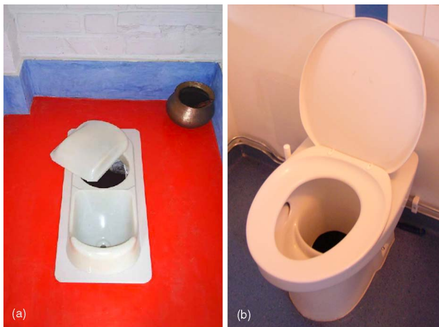
Fig. 5. (a) A urine-diverting dry squat toilet from India (photo: S.Vishwanath www.rainwaterclub.org ); (b) a urine-diverting dry toilet from Sweden (photo: Dana Cordell).
